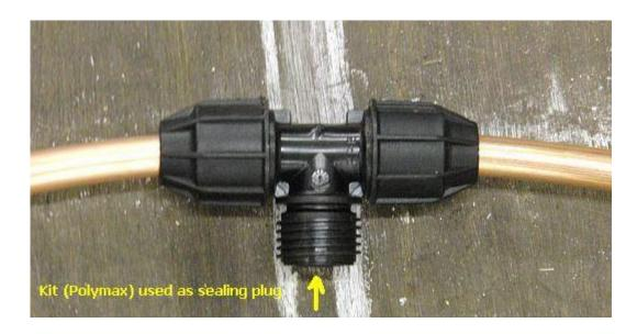
The plastic T connector, who is mounted on the standpipe, is sealed with suitable kit such as Polymax to avoid any water leakage or
