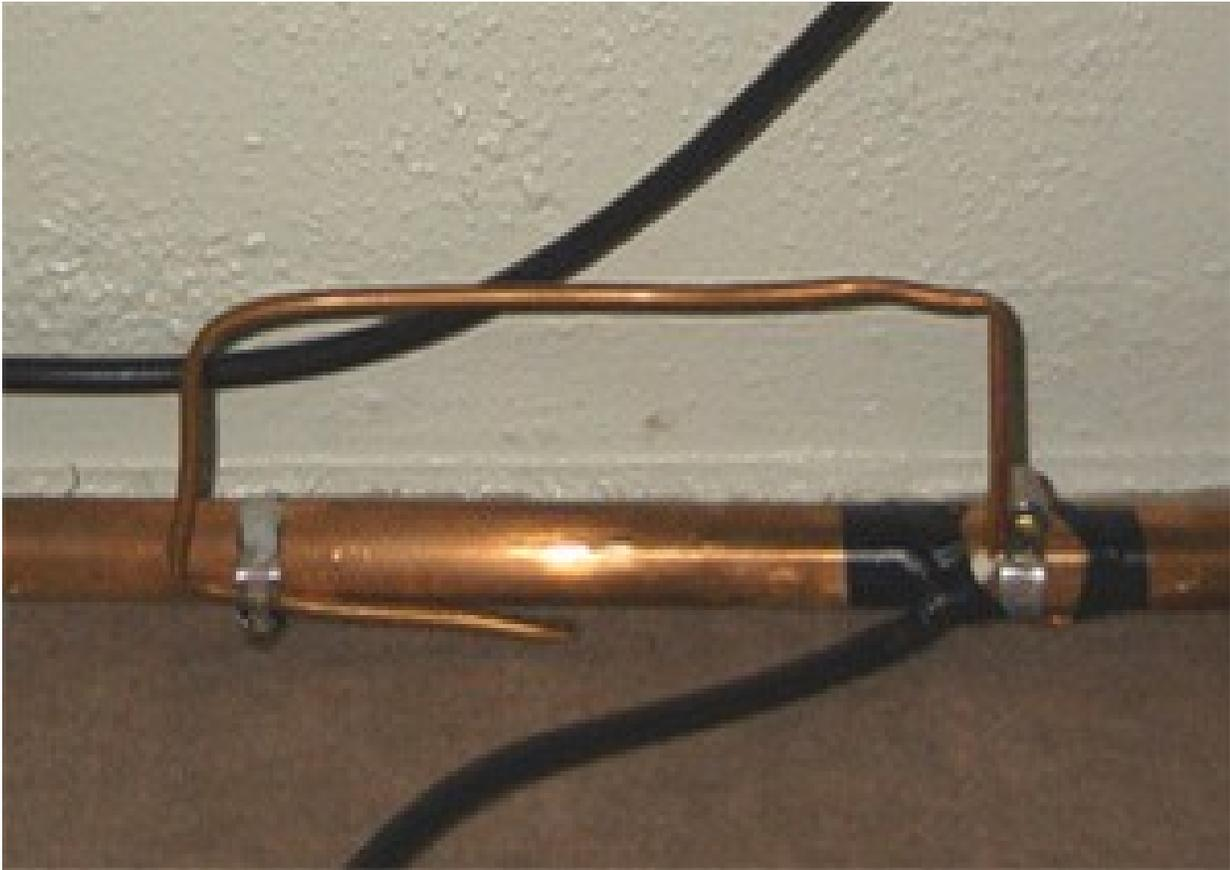
4. Finishing the Feed: Take your second radiator clamp and put it on the loop loosely on one side 5 or six inches from either side of the loop. It doesn't matter which side. Now place your thick copper wire, or think copper pipe through the radiator clamp off the one side and tighten it so it's secure, but you can still move it. It isn't important if you have too much wire or pipe, you may need it later, so don't bend it too much just yet.
