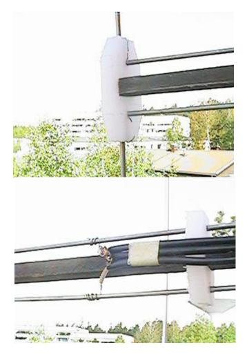
I have not shown the dimensions of the cut blocks but the inserts in the first picture show you exactly how they are formed. It all depends upon what size wooden mounting boom you have. It could of course be metal, but I had a bit of wood sitting doing nothing on the balcony. The only important bit is that the stub should be 1/4-wave in length, not counting the shorted (folded) end.
