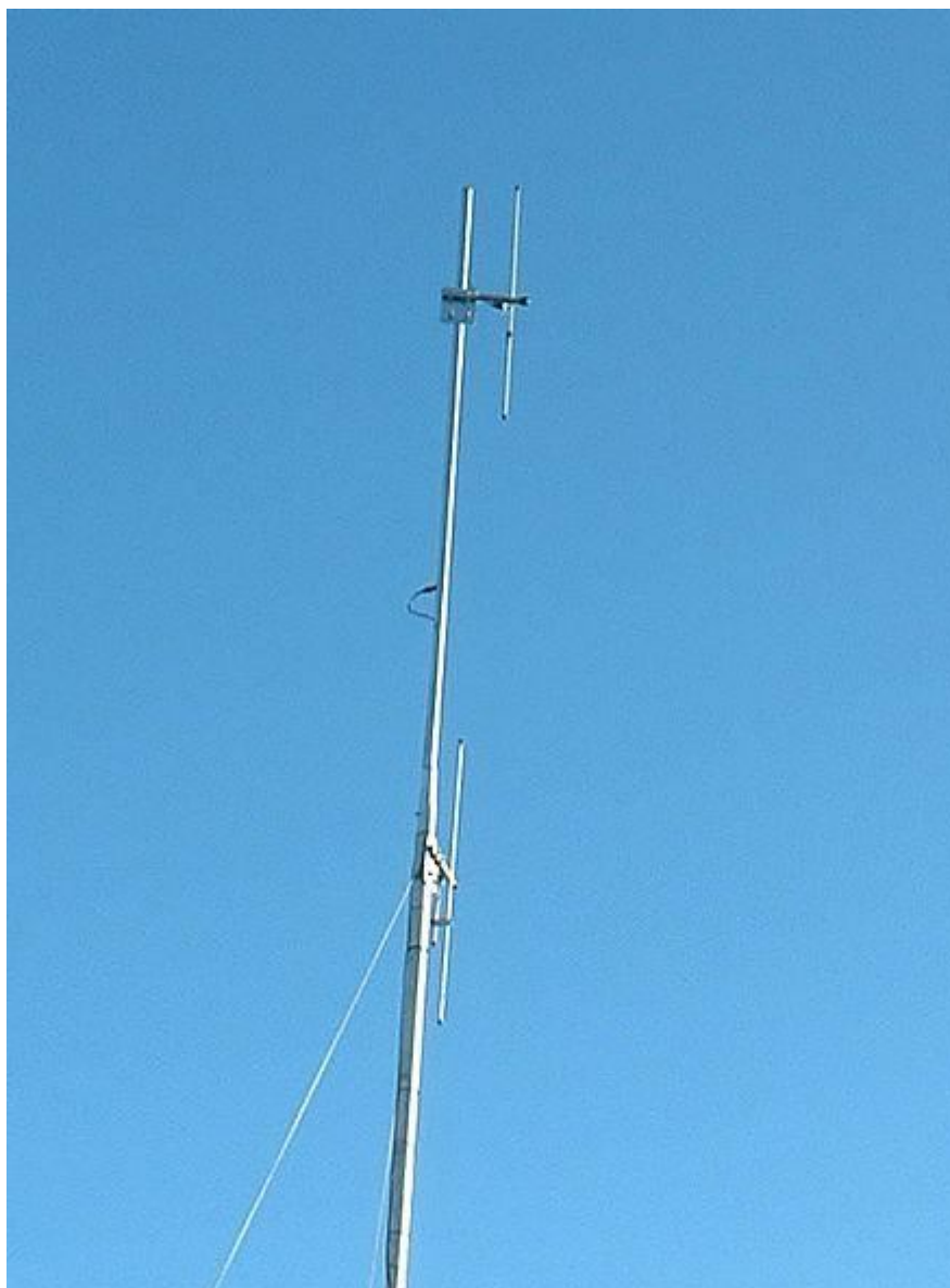
Photo: Co-phased Dip-Yag's on the mast.
