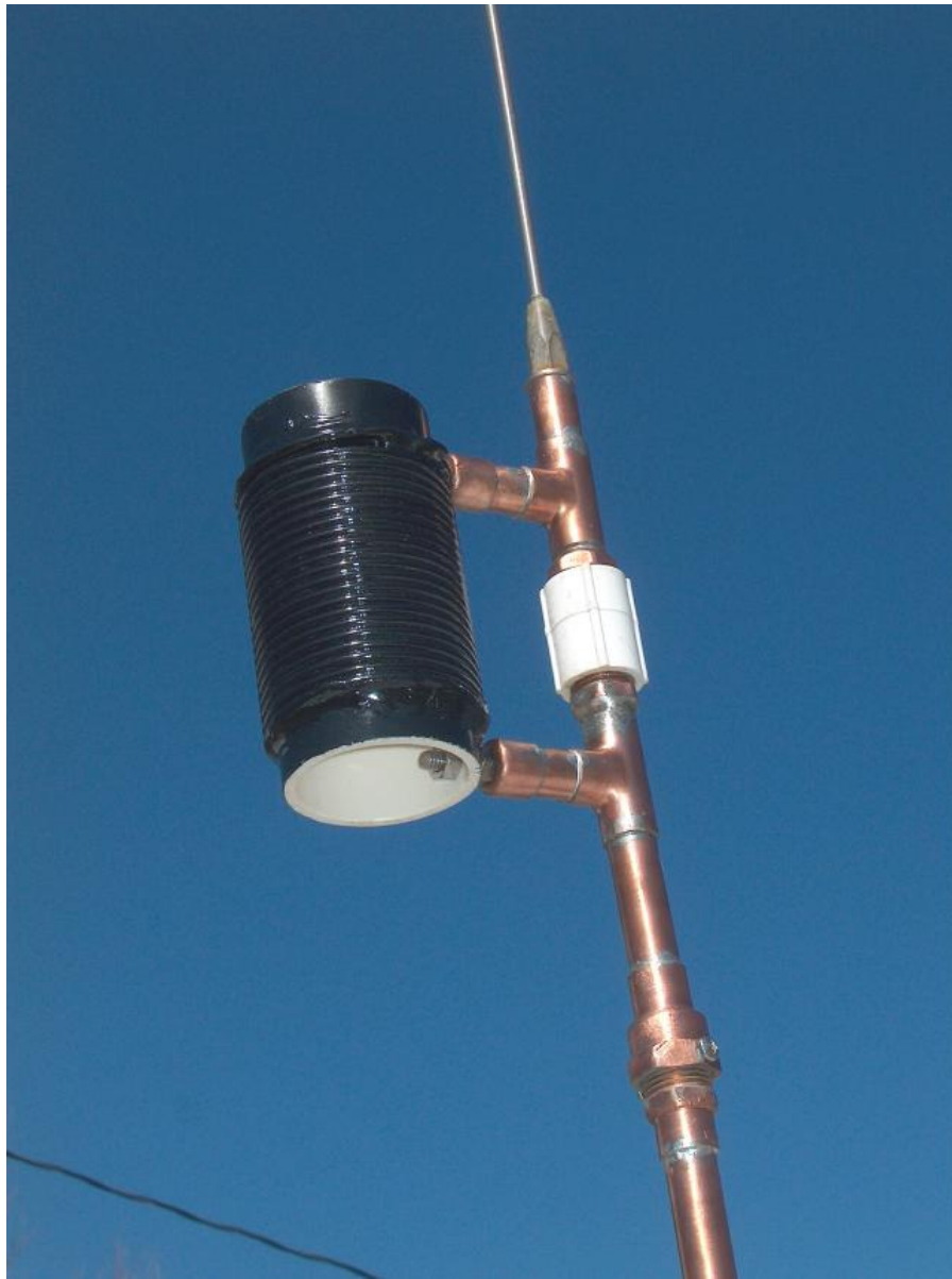
The 40 Meter loading coil in place on the antenna.
