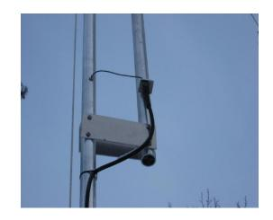
The coax was routed down the main mast to a coax relay so that a single coax feedline could be used with the antenna. A small 12-vdc relay switches 115-vac to the coax relay. An extension cord provides 115-vac to the relay box and a run of No. 16 speaker wire provides 12-volt control from the "radio shack".
