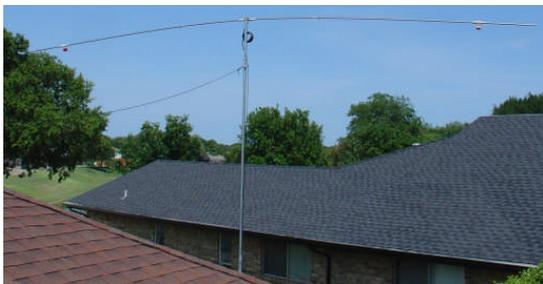
Photo E: Completed 17/12M trap dipole
