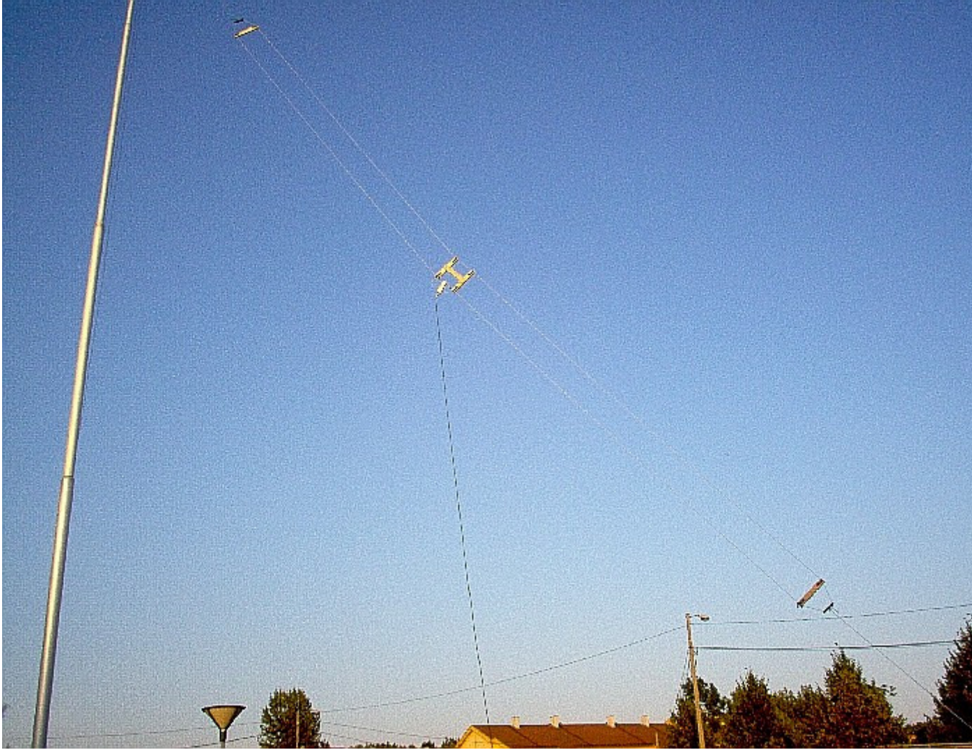
The 20 m folded dipole as a Slope.
